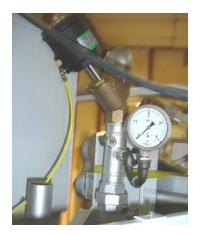
Steam inlet DN 50, pressure regulation with manometer
